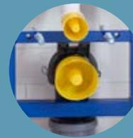
**7** Protective plugs fitted to protect the connections during installation.
