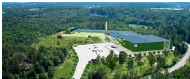
THE NEW FACTORY BUILDING IS SCHEDULED FOR COMPLETION IN 2014.
